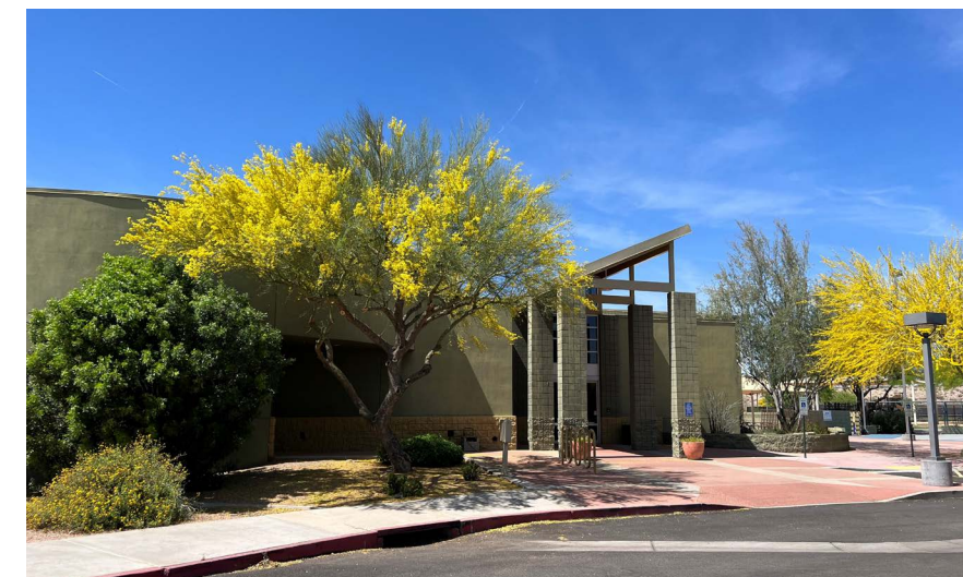
Local community center
